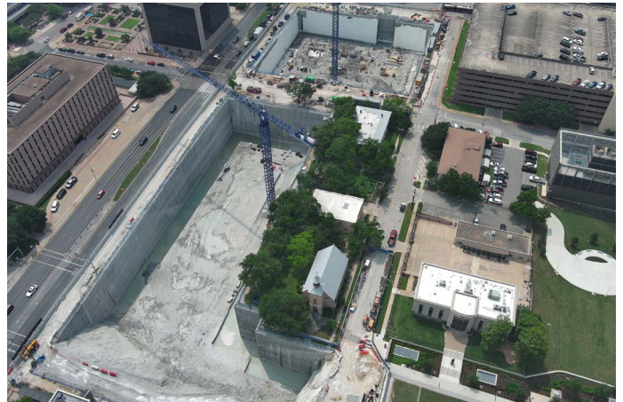
Excavation nearing completion, May 2024.
