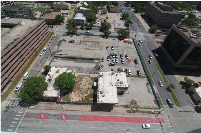
At the beginning of the project, preparing for demolition, March 2023.
