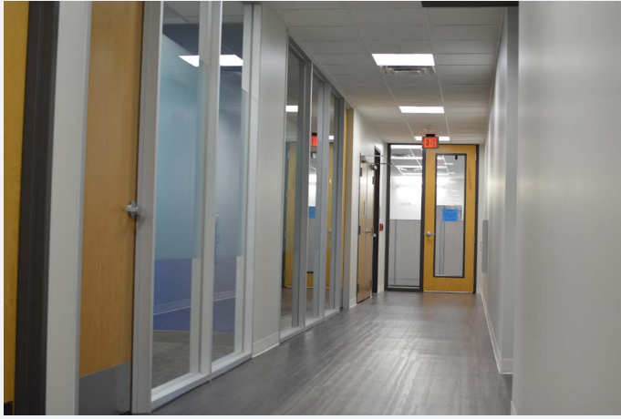
Renovation work at the Lyndon B. Johnson State Office Building.
