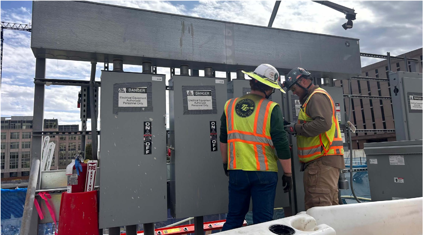
Tumlinson working on Phase II of the Capitol Complex Project. Photo courtesy of JE Dunn Superintendent Mike Hamline.
