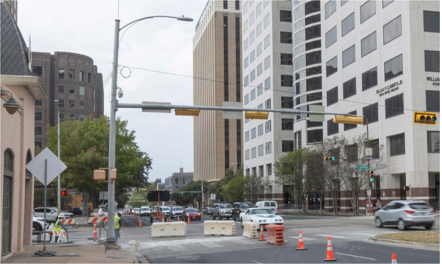
Traffic barriers for temporary lane closures on 15th Street.
